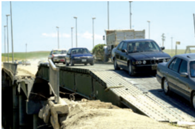
Dry support bridge (DSB)
