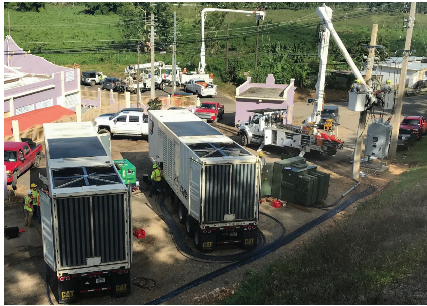
Arecibo, Puerto Rico – The U.S. Army Corps of Engineers Task Force Power Restoration assists with the installation of a microgrid in Arecibo, Puerto Rico, 30 January 2018. Potentially 250 households and infrastructure in Arecibo will be powered once the microgrid is activated. The USACE installed seven active microgrids around the island (Photo by Robert DeDeaux/USACE Public Affairs).
