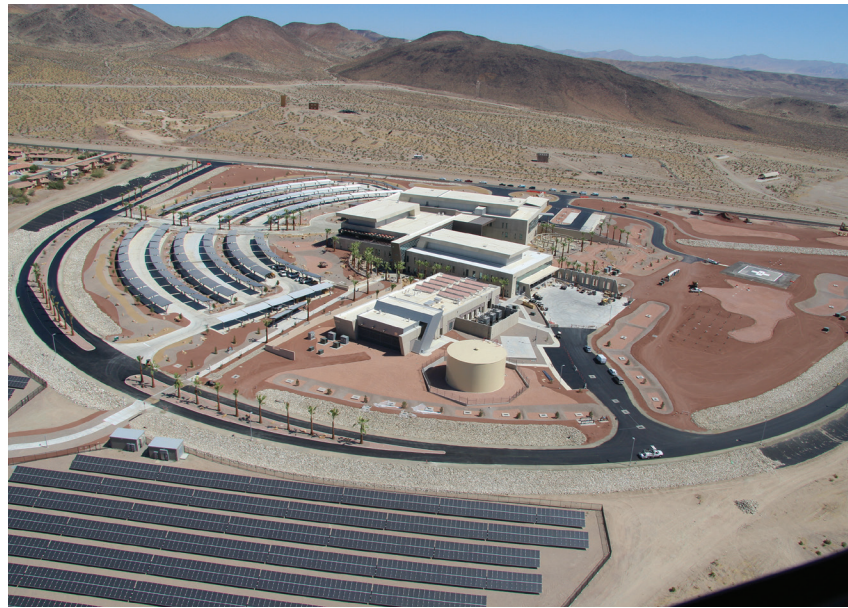
The new Weed Army Community Hospital, as seen in this June 2017 photo, is DoD’s first Leadership in Energy and Environmental Design (LEED)-Platinum, carbon-neutral medical facility built in the United States. It generates all of the energy it needs by solar power and other renewable energy systems. It is one of three LEED-Platinum medical facilities built in the United States, but the only one built for DoD (Photo by Brooks Hubbard/USACE).
