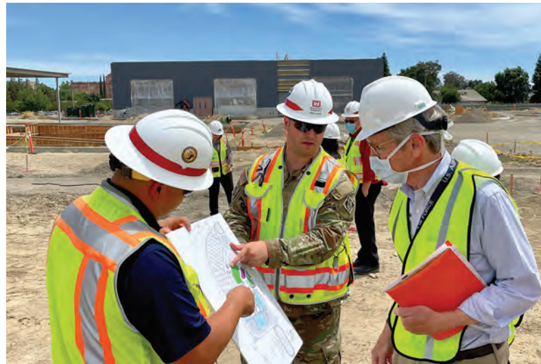
Major Nicholas Yager, a project manager with the U.S. Army Corps of Engineers Sacramento District, and Earl Chow, left, a construction engineer with the Sacramento District, explain the layout of the future Veterans Affairs (VA) Stockton Community Based Outpatient Clinic to Dr. William Cahill, chief of staff for the VA Northern California Health Care System, 8 June 2022, in Stockton, California. The USACE Sacramento District has been constructing the clinic for more than two years, with plans to build additional facilities including a Community Living Center and Engineering Logistics Building (U.S. Army photo by Jeremy Croft).
