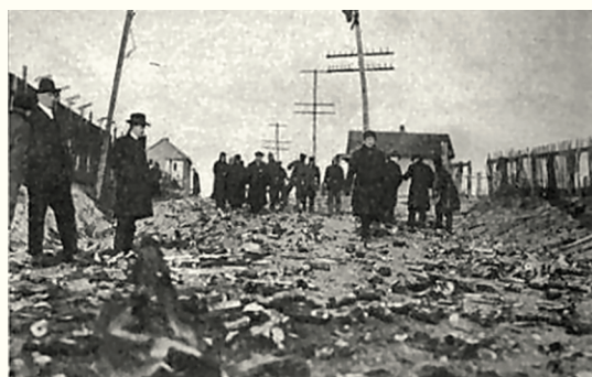
Figure 12. Canadian Car and Foundry Company's Plant, Kingsland, New Jersey, after the fire and explosions (Photo 1917 International Film Service, Inc.).
