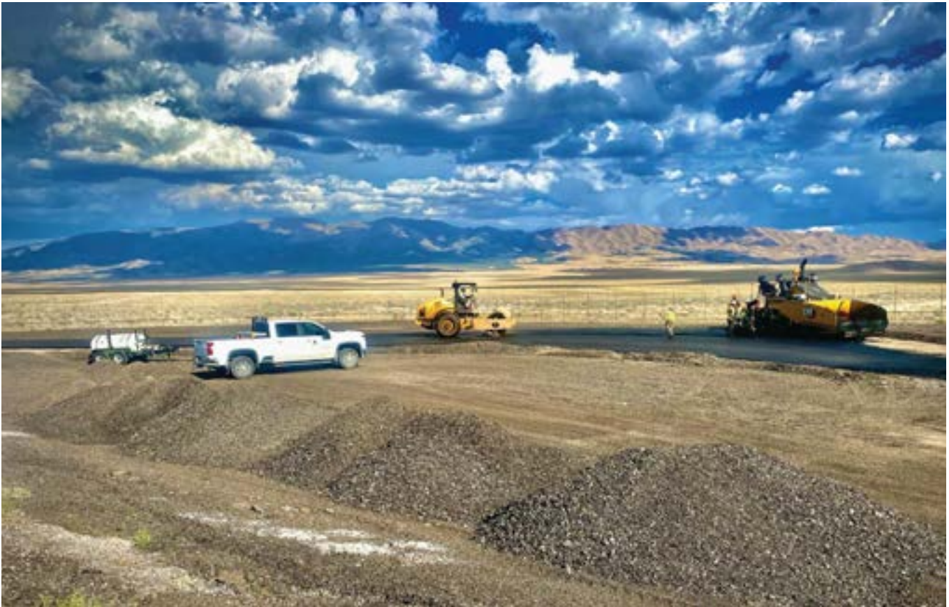
Repaving work is underway at Dugway Proving Ground, Utah.
