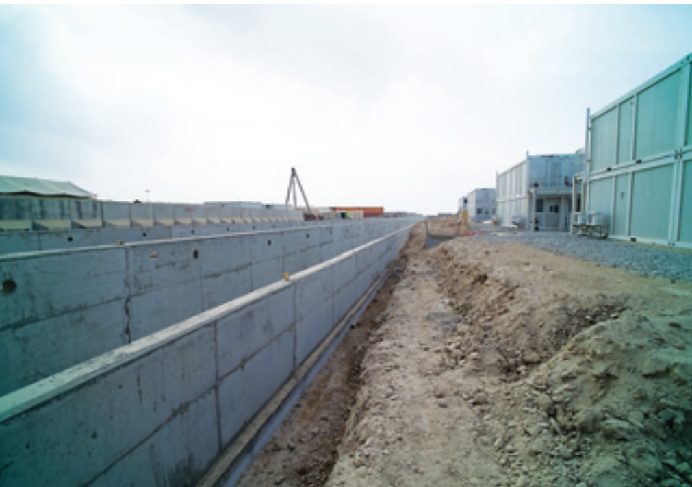
To expand living space, a concrete channel diverts the natural flow of a wadi that runs through NATO's Kandahar base.
