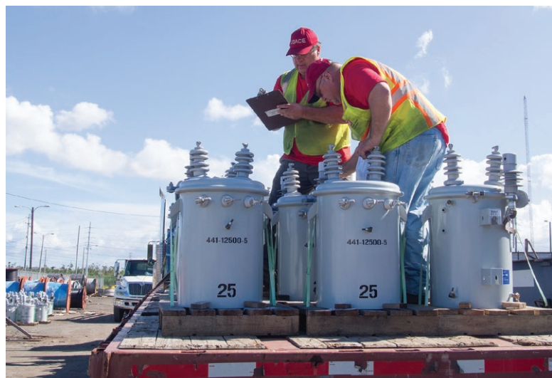
Quality Assurance personnel with the USACE, Taskforce Power Restoration, Andrew Imig and Micheal Nordhaus inspect and inventory KVA-25 transformers as they arrive in the Palo Seco Warehouse and Laydown yard on 20 January 2018, in San Juan Puerto Rico. The transformers were then transported to the Palo Seco warehouse for distribution to the local vendors. Upon arrival, after inspection and inventory, they were immediately sent the Puerto Rico Electric Power Authority office in Rio Grande, Puerto Rico (U.S. Army photo by Staff Sergeant Eric W. Jones).
